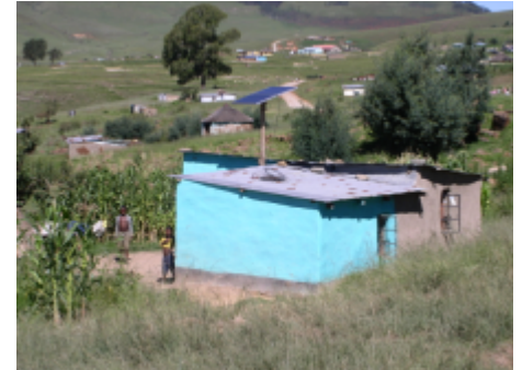
Fieldtest in a village with Solar Home Systems in South Africa
